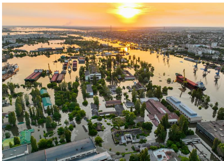
Fig.2. The massive floods after the destruction of the Nova Kahovka dam in Kherson / (photo source: Shutterstock) [12]
